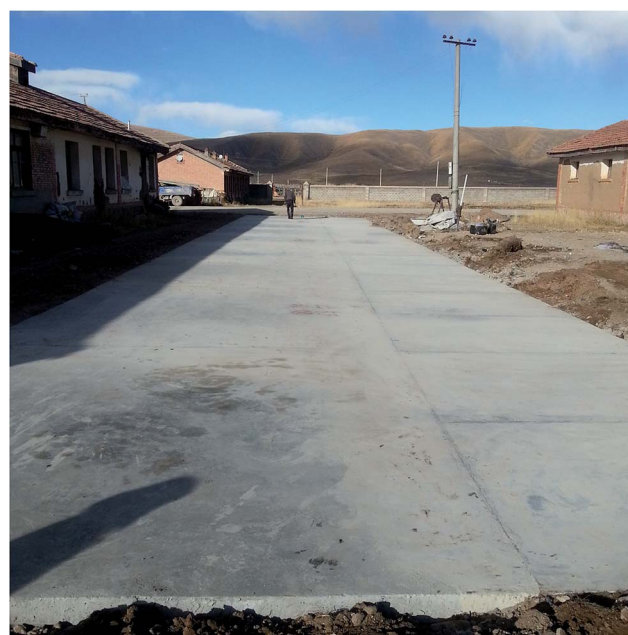
Fig. 17 Field test section.
