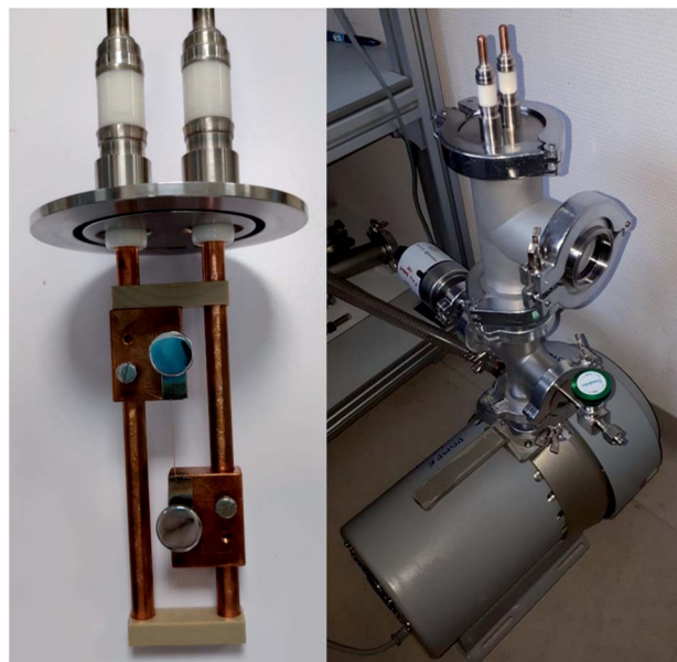
Fig. 2 Setup used for ampacity measurements. The sample line is mounted on a support allowing to control the distance between the two electrodes (left). This support is inserted in a pressure controlled chamber (right).
