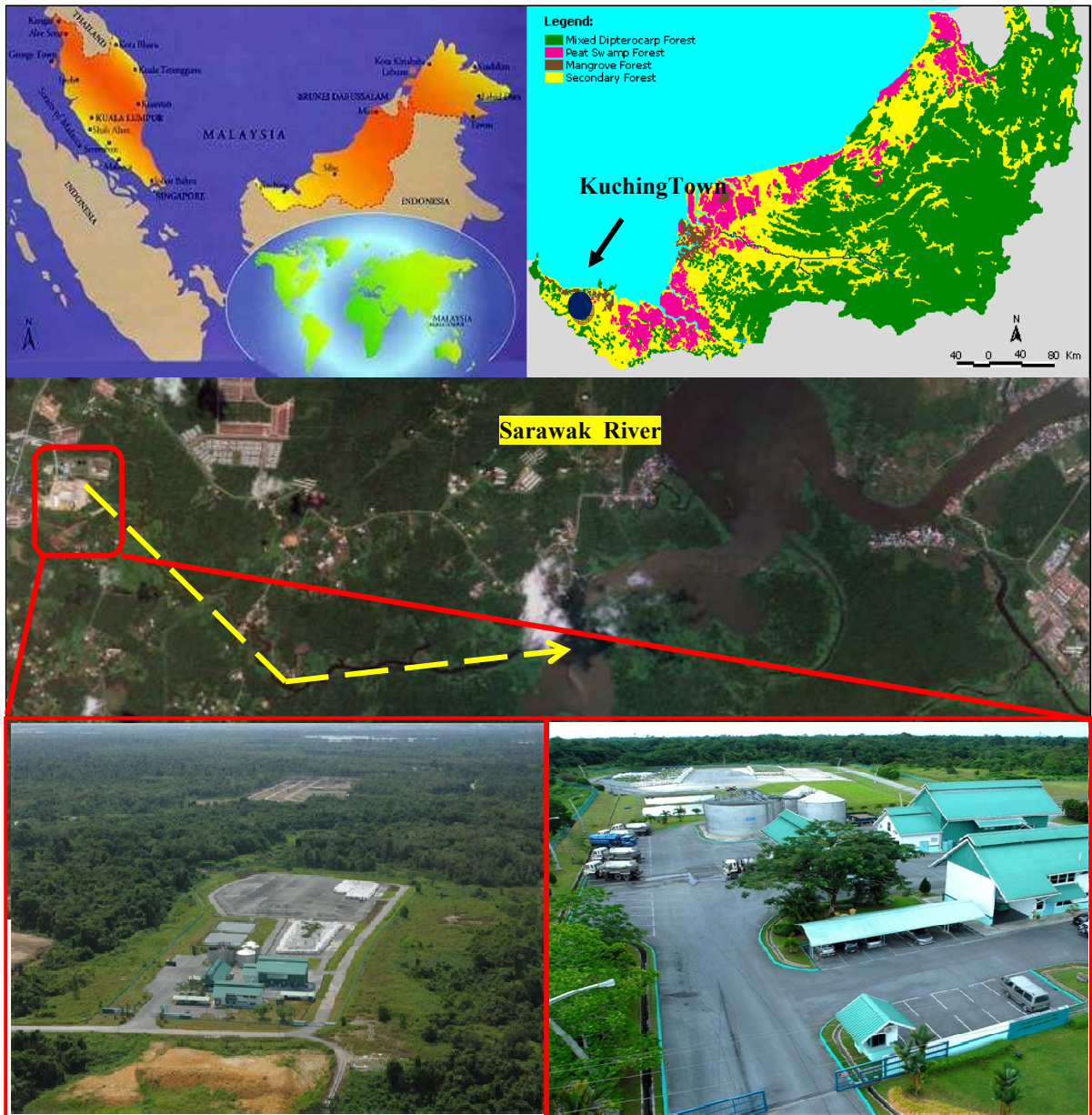
Fig. 1: Septic sludge treatment plant in Matang, Kuching, Sarawak.
