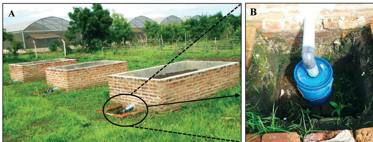
Fig. 1 Faecal sludge treatment system in Kining'ina, Tanzania. A. Three solar drying beds for faecal sludge treatment B. Faecal sludge leachate outlet and 20 L collection bucket.
